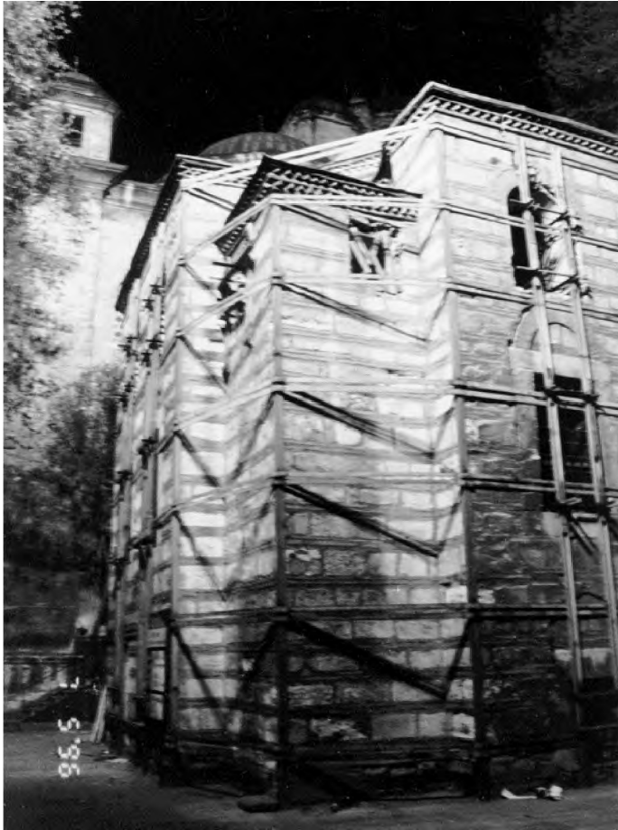
Fig. 12.57. Close-up view of the Church of Mehmed II the Conqueror. The building is gradually falling apart. To protect it, it was pulled together from all sides with iron reinforcement. Photo of 1996.
