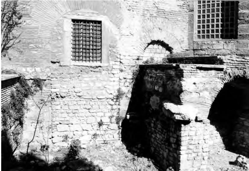
Fig. 12.16. Wall of the temple of St. Irene in Istanbul. The temple has sunk deep into the ground. Today its lower part has been excavated and is now visible. Photo of 1996.
