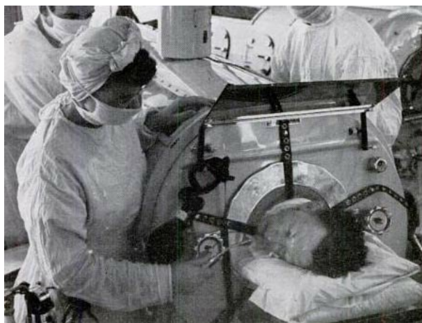
Photo 12.3: Iron lung encases 27-year-old Boyce Rash whose respiratory muscles have been paralyzed. Breathing function is so impaired that a mechanical apparatus is required to force air in and out of the patient's lungs. Seven iron lungs were shipped to Hickory, two of them from Boston. John Bryan, 8, uses oxygen inhalator. It feeds oxygen to nose of patient who has difficulty in breathing normally. Most severe cases involve paralysis of respiratory muscles. Tube extending from mouth collect saliva which boy cannot swallow because of paralyzed throat muscles. (1943)
